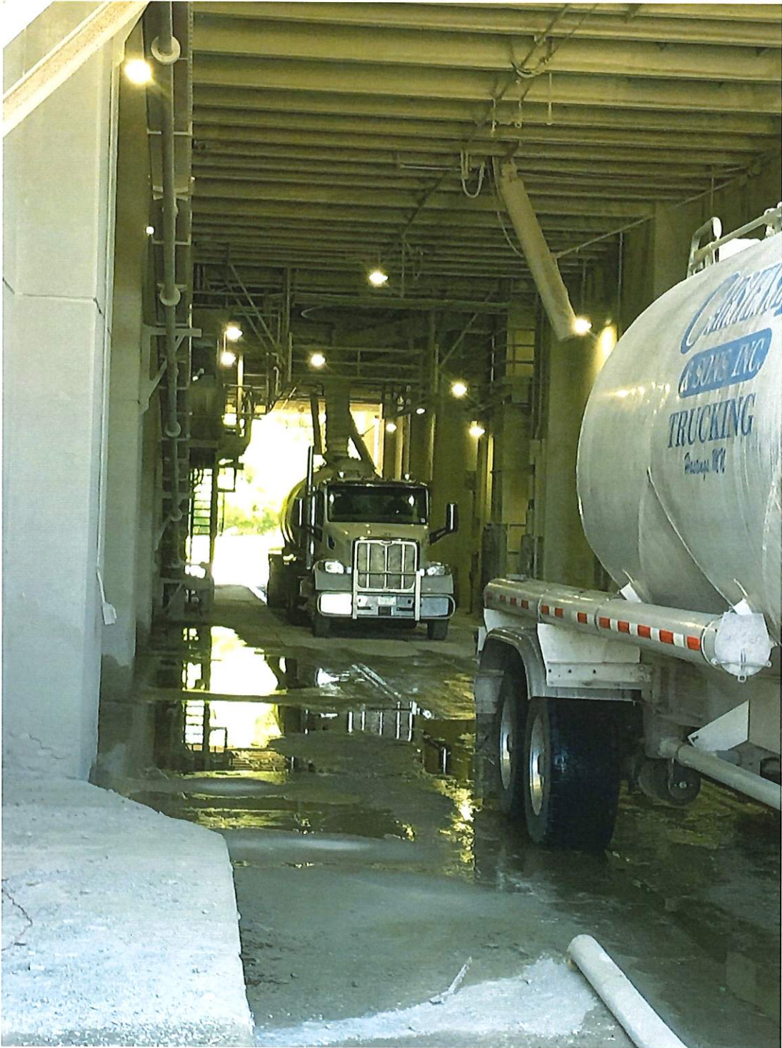
This photo was taken in the 30-bay mentioned in the complaint. It illustrated the visibility conditions from entrance to exit at the time of my investigation.
