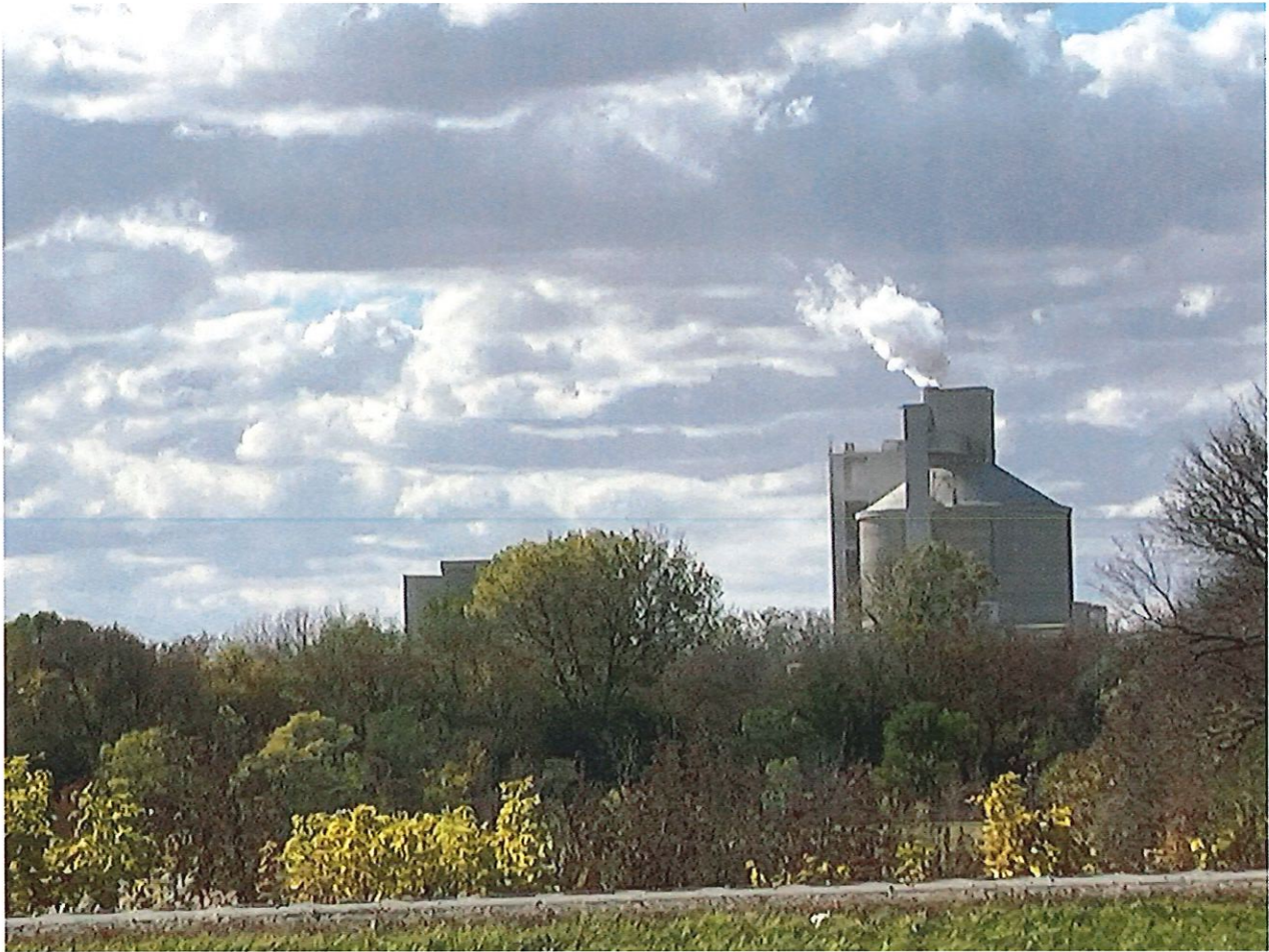
Photo 1: Emissions from Heidelberg Materials on the afternoon of October 18, 2023. Only the steam plume was visible. Photo by David Knoll, FO2 (looking west).
