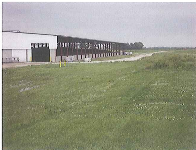
West wall of manure containment building after clean up
