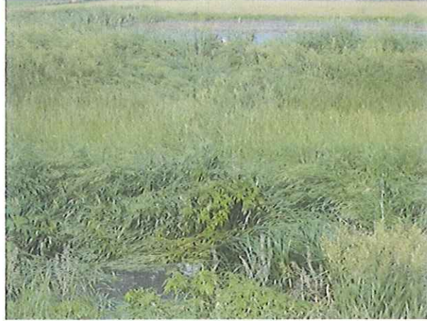
Storm water basin and discharge pipe
