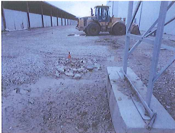
Storm water drain between manure building and production buildings.
