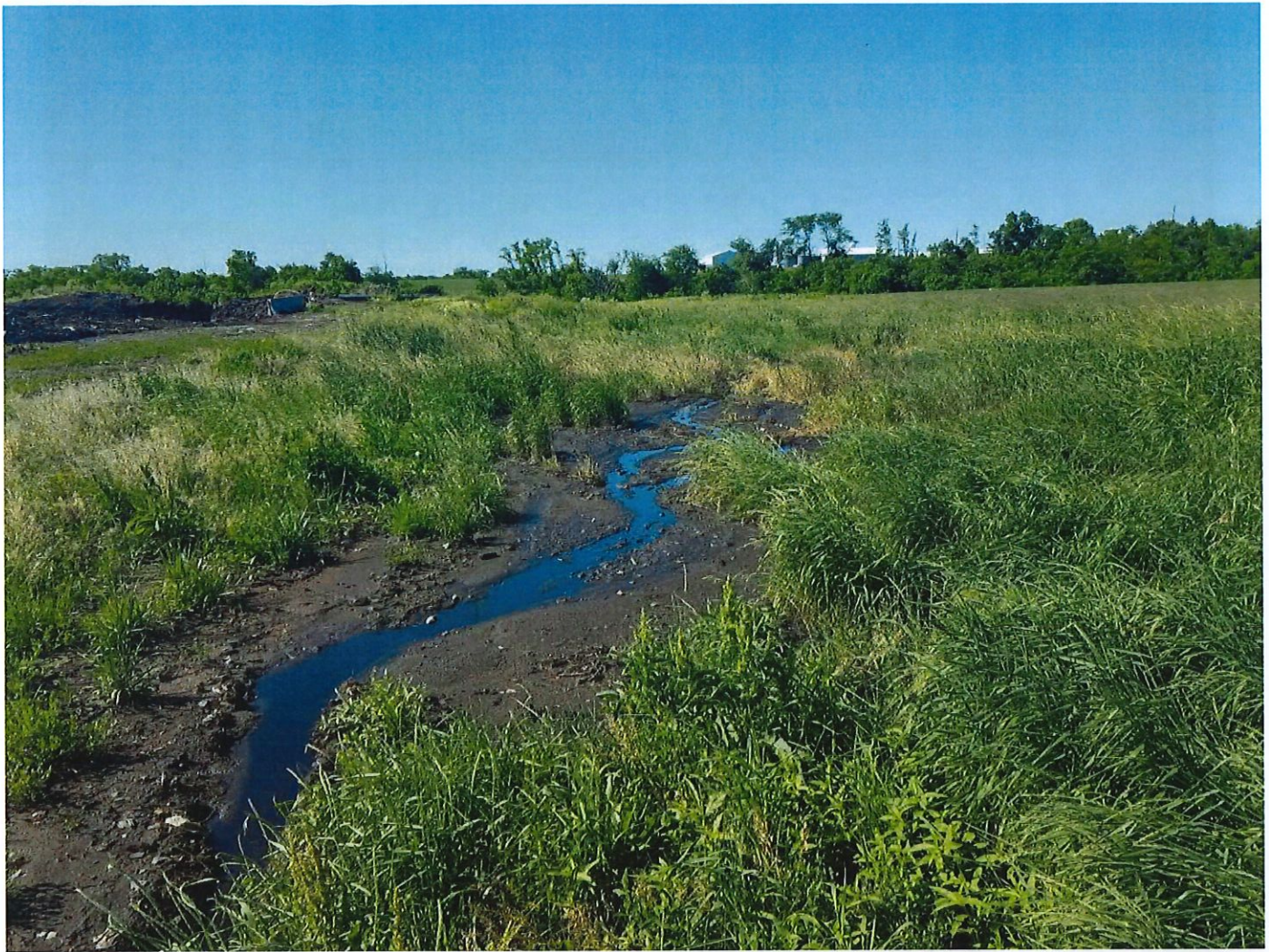
Picture 1. Taken 6/11/20. Looking south from northwest corner of the compost pad. Leachate can be seen off the west edge of the pad, flowing south. This leachate enters a drainageway, flows around the west lagoon, and enters the tributary of Palestine Creek, as seen in picture 2.
