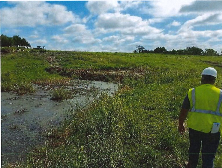
Pictures 7 & 8. Hay bale and earth berms are in place downslope of compost fill operation.
