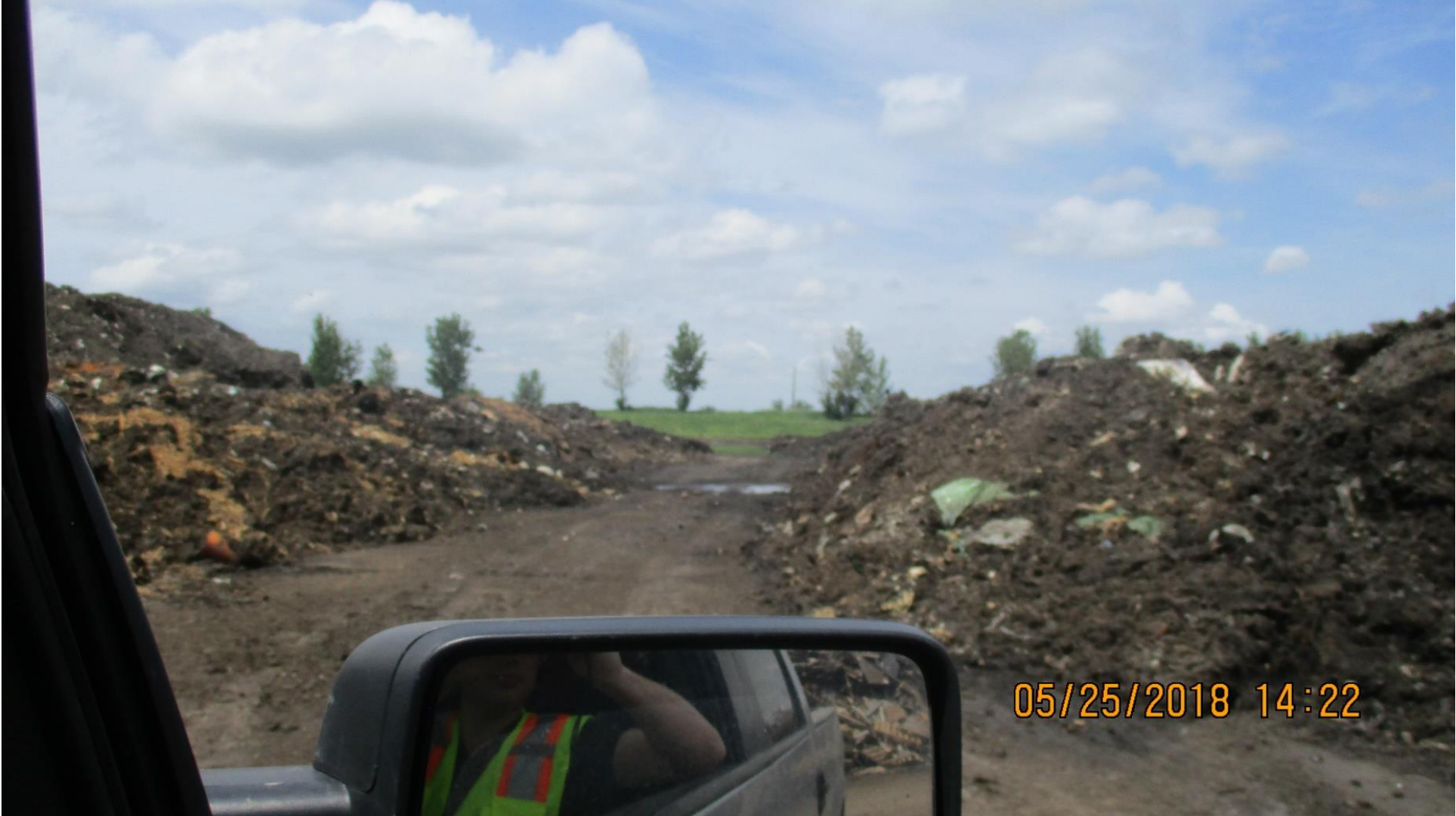
Chamness Technology, Inc. – View of central portion of composting pad looking north
