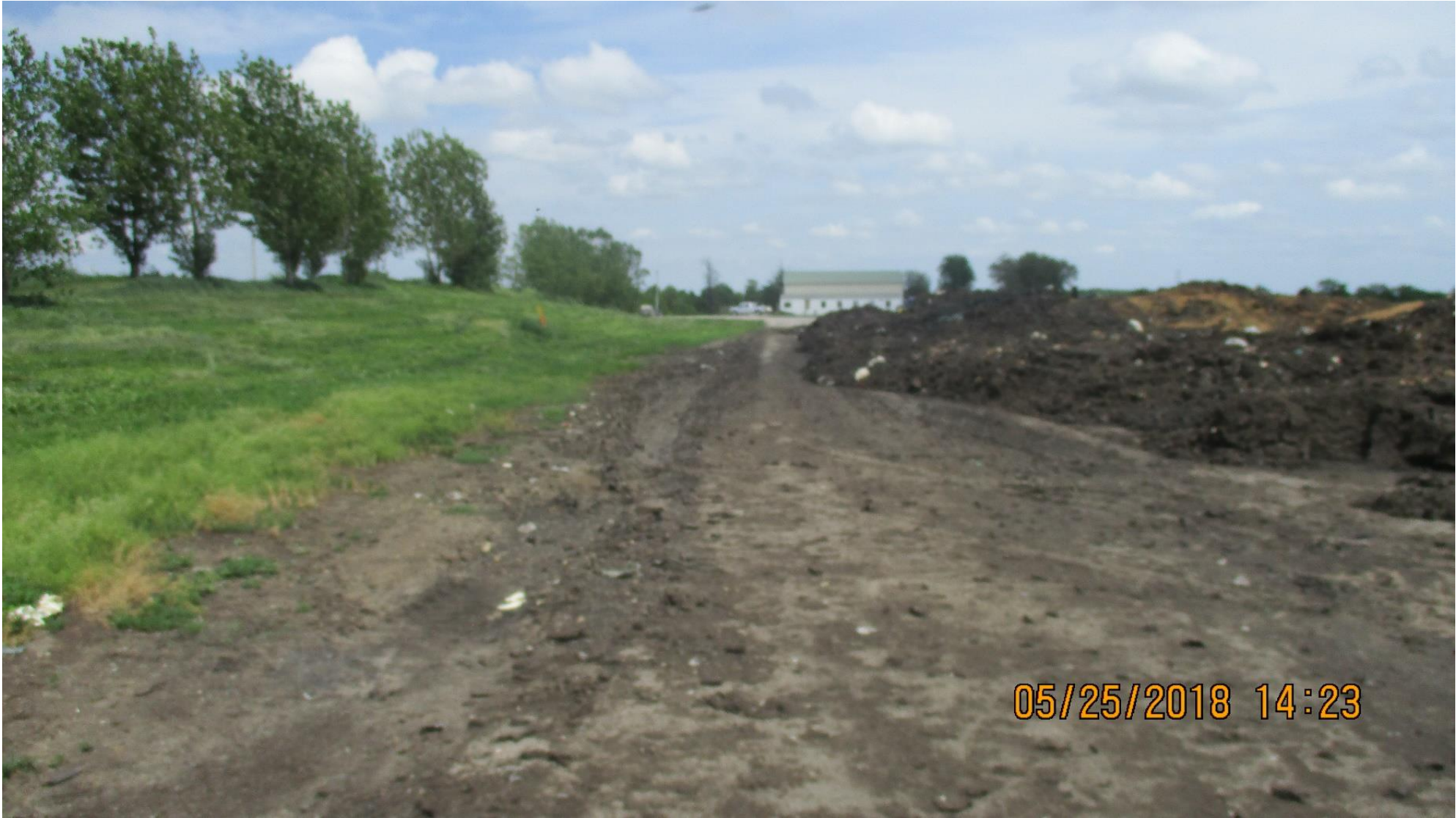
Chamness Technology, Inc. – View of eastern portion of composting pad looking east
