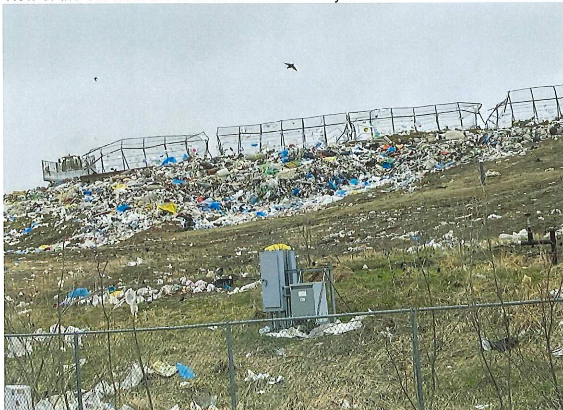
View from Northwest of the facility. Solid waste seen outside of the wind screens.
