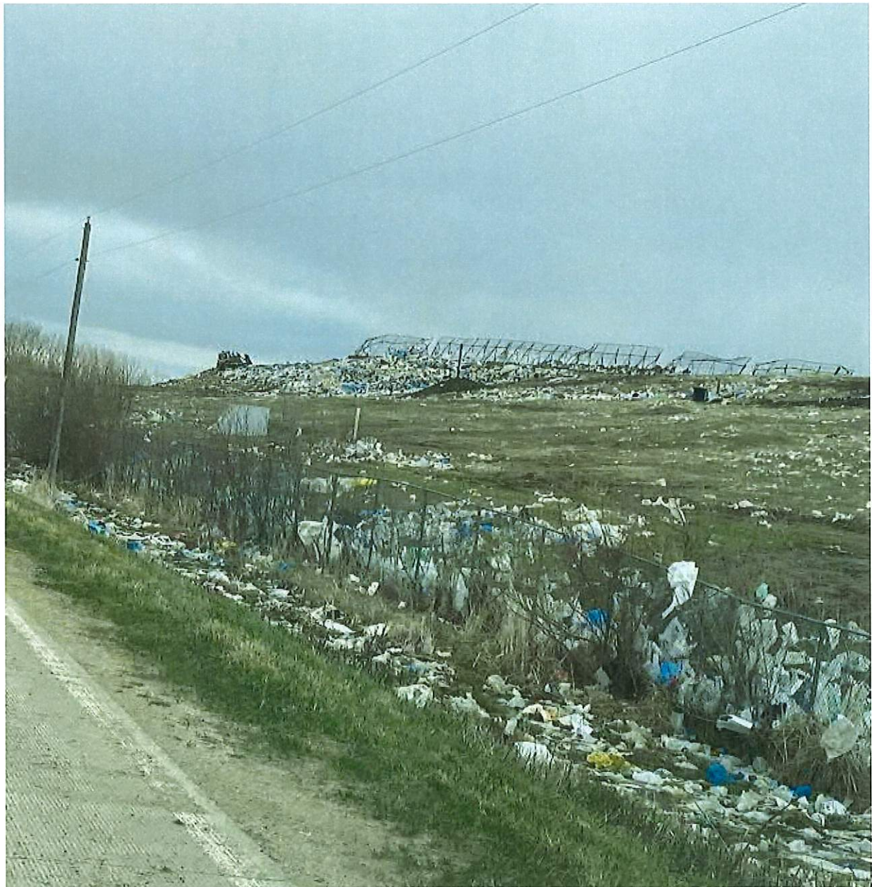
View of the cell and ditch from the north/northwest of the facility.
