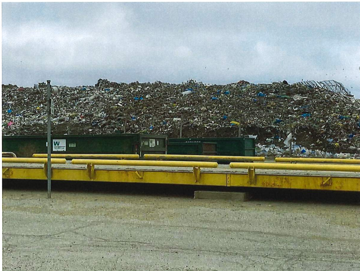
The cell seen from the office of the facility. No cover down slope.
