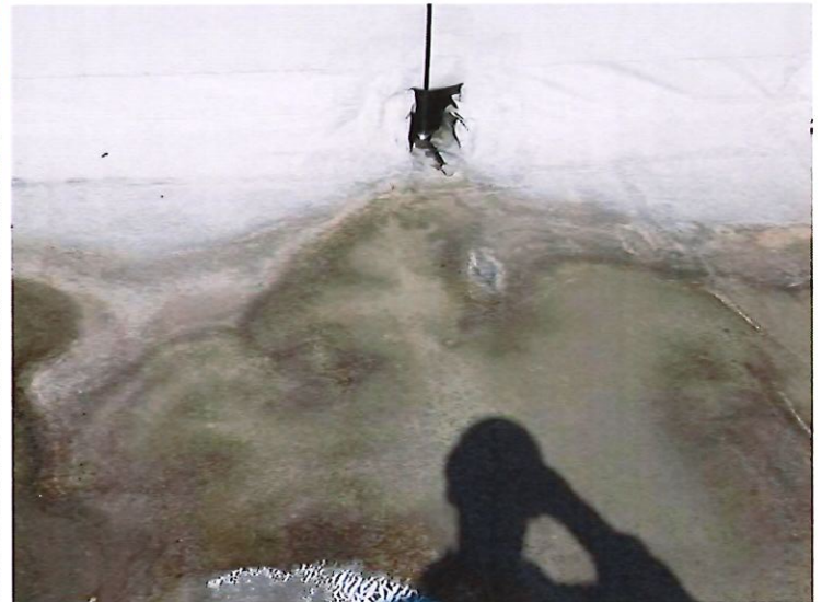
View looking west at roof drain inlet in the northwest corner of the roof near EP-12.
