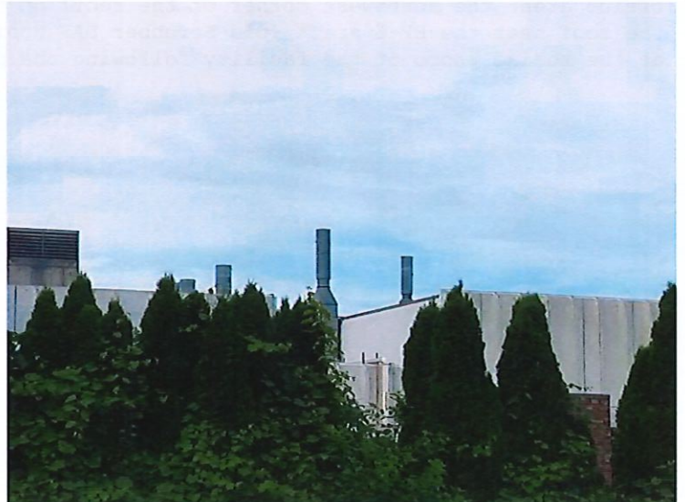
View looking south at the facility from the adjacent Super 8 facility to the north.
