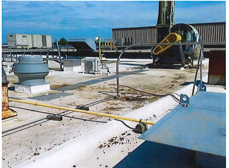
View looking north-northwest at materials on the roof near EP-6 - Old Scrubber Stack (upper right).
