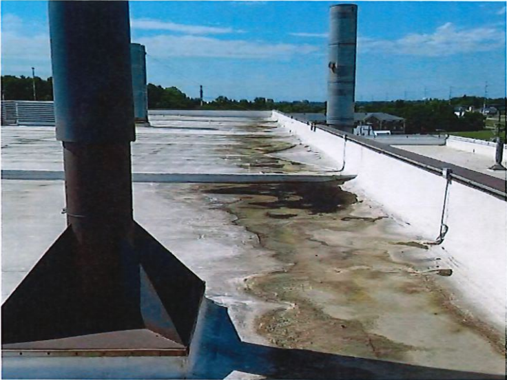
View looking south from EP-12 (left stack) along the west edge of the roofline by EP-12. EP-18 and EP-19 can be seen in the background (from left to right, respectively).
