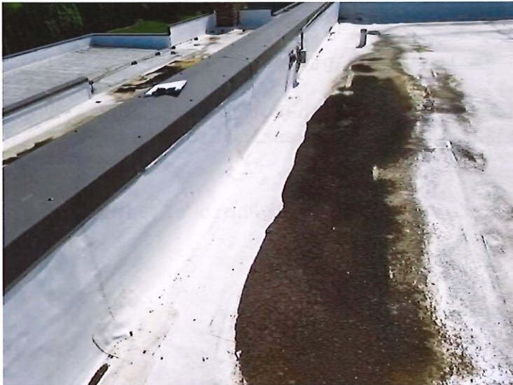
View looking east along the north edge of the roof over the Boiler Room.
