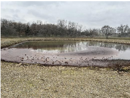
East lagoon full of sludge.
