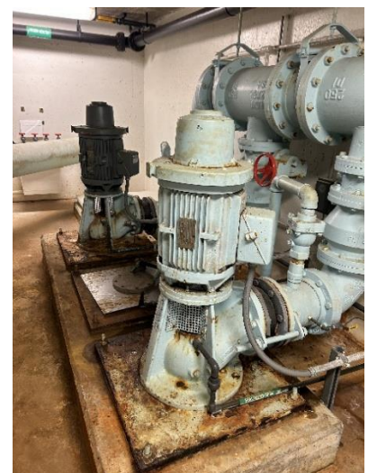
Transfer pump #5 removed.
