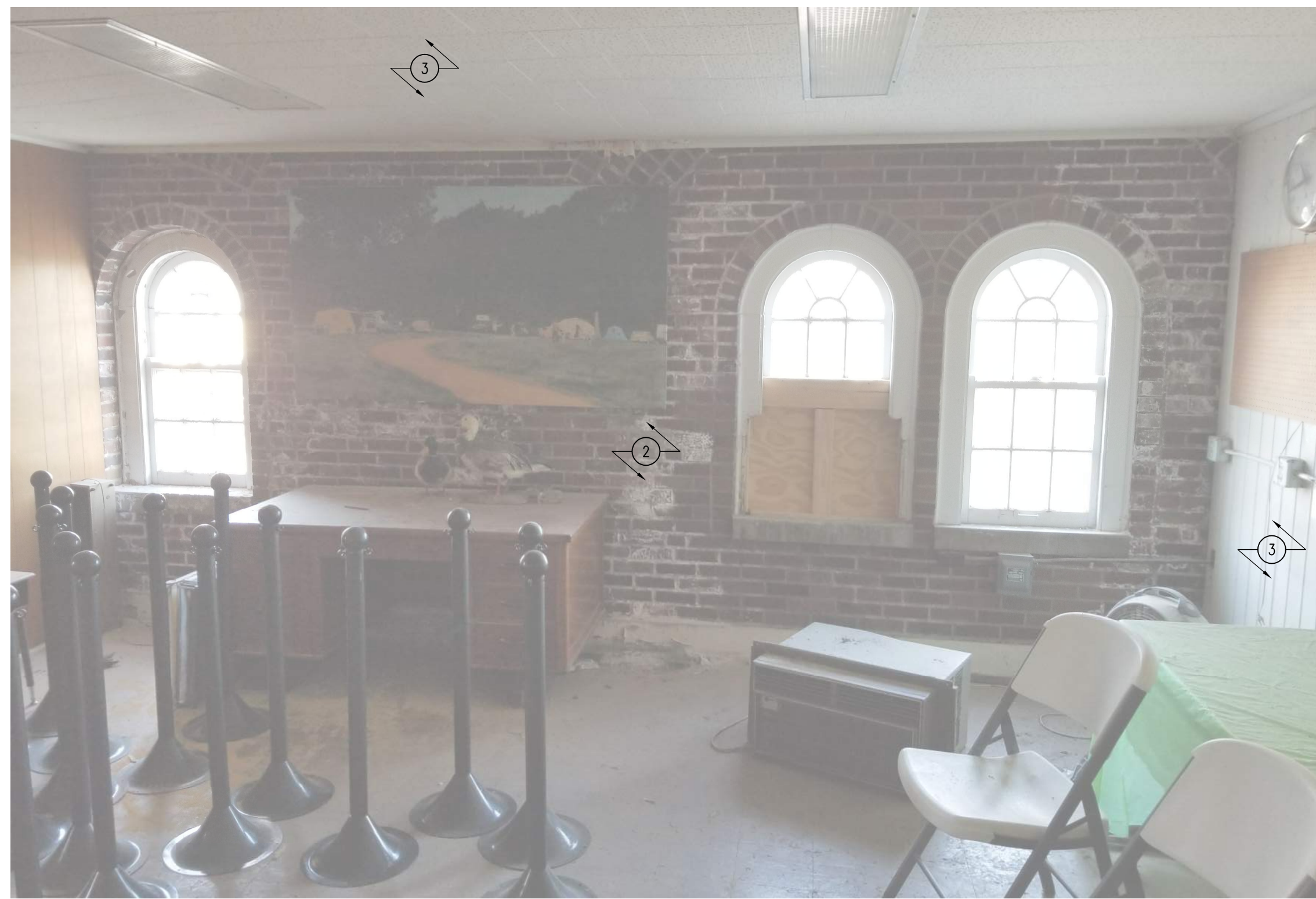
01 DNR PAVILION – UPSTAIRS EXISTING CONDITIONS SCALE: NTS
