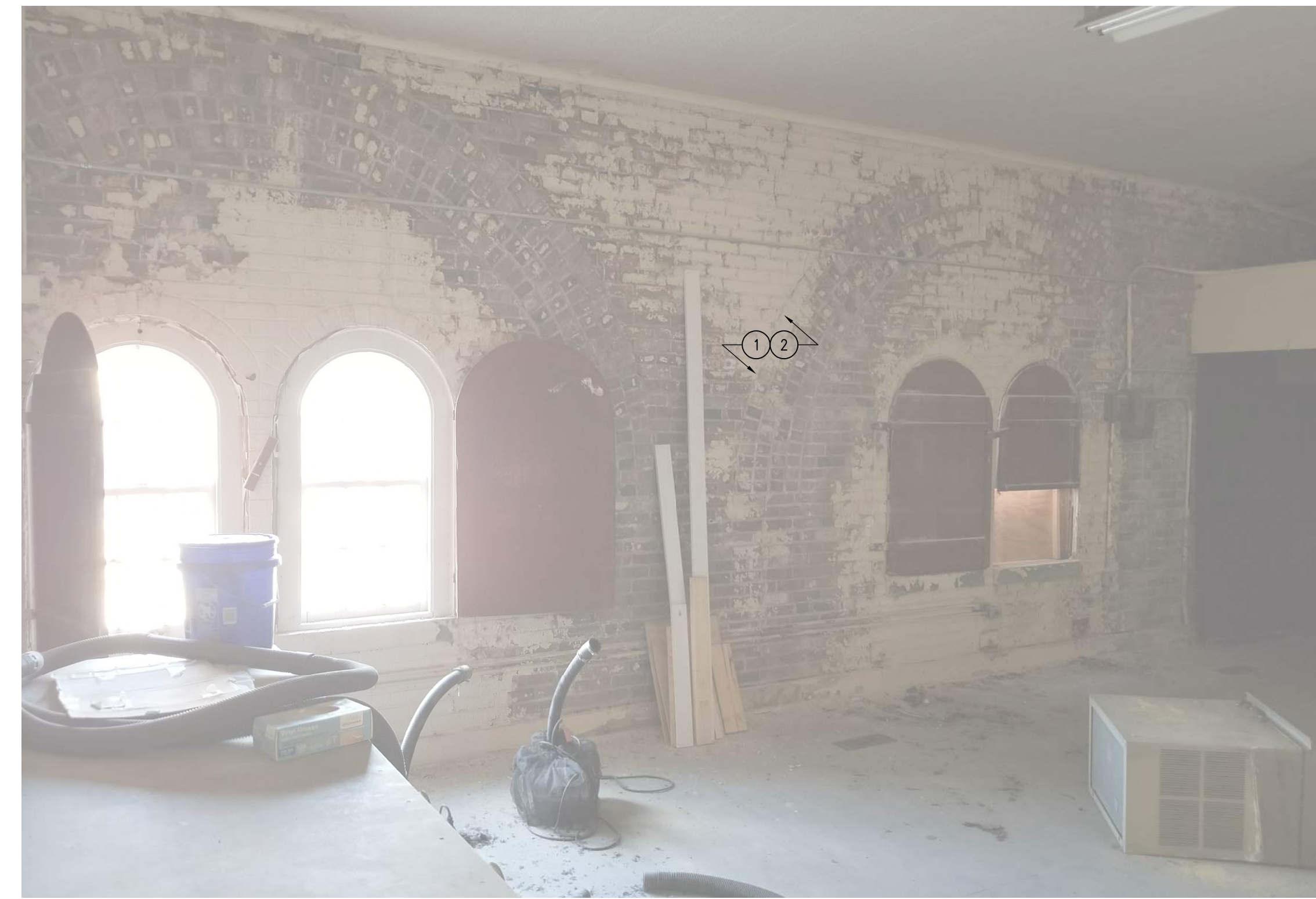
03 DNR PAVILION – UPSTAIRS EXISTING CONDITIONS SCALE: NTS
