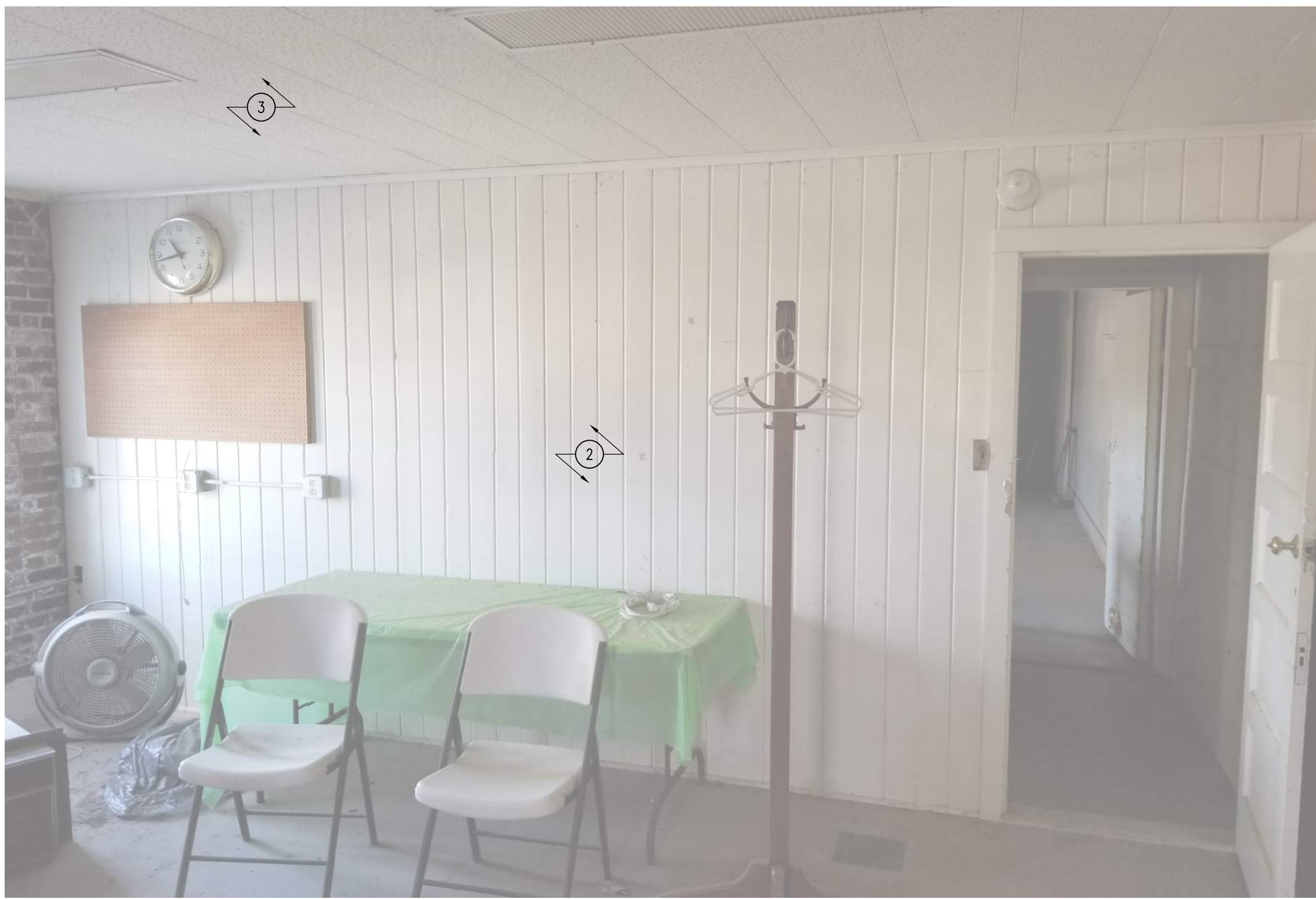
02 DNR PAVILION – UPSTAIRS EXISTING CONDITIONS SCALE: NTS
