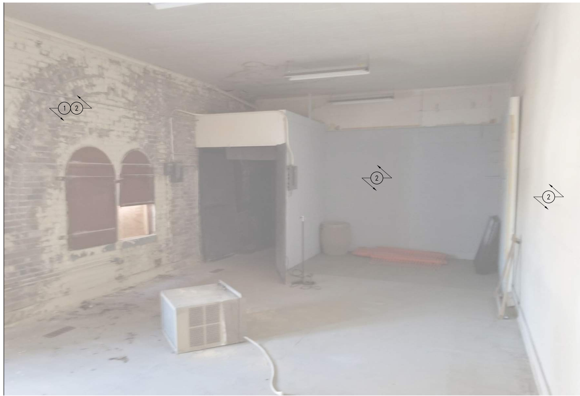
04 DNR PAVILION – UPSTAIRS EXISTING CONDITIONS SCALE: NTS
