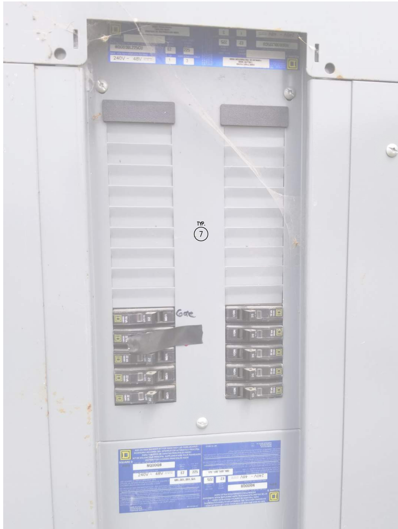
03 PHOTO - ELECTRICAL SUBPANEL SCALE: NTS
