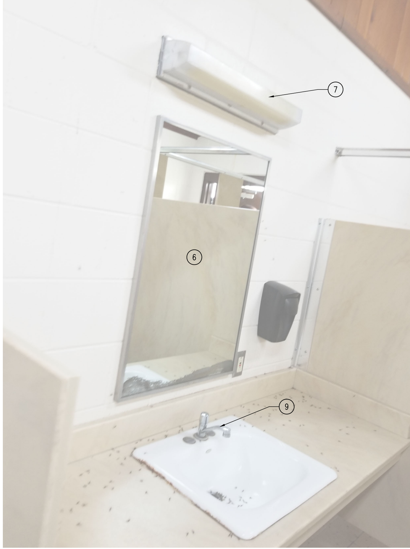
02 PHOTO – BEACH RESTROOM EXISTING CONDITIONS SCALE: NTS
