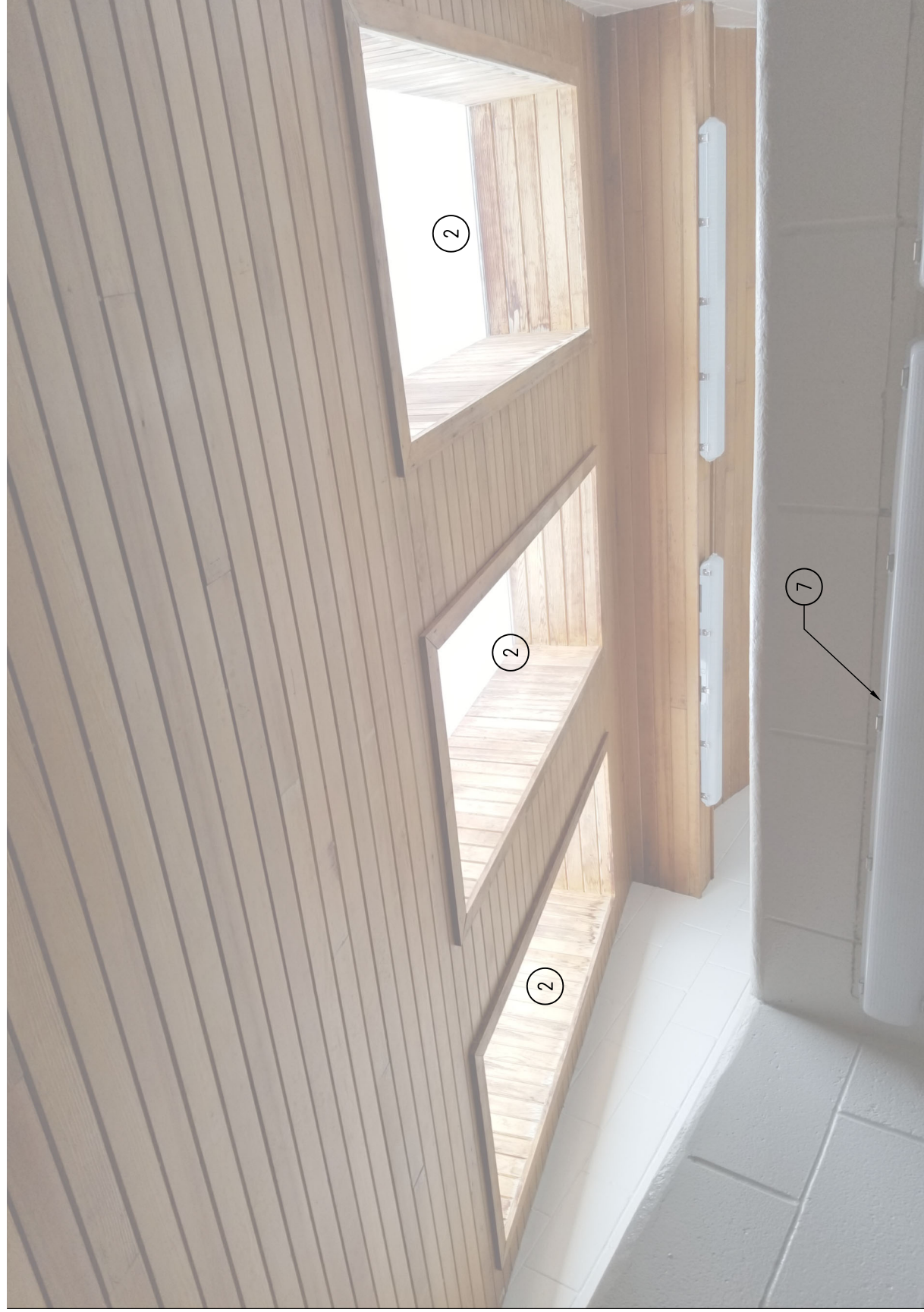
01 PHOTO – INTERIOR EXISTING CONDITIONS
