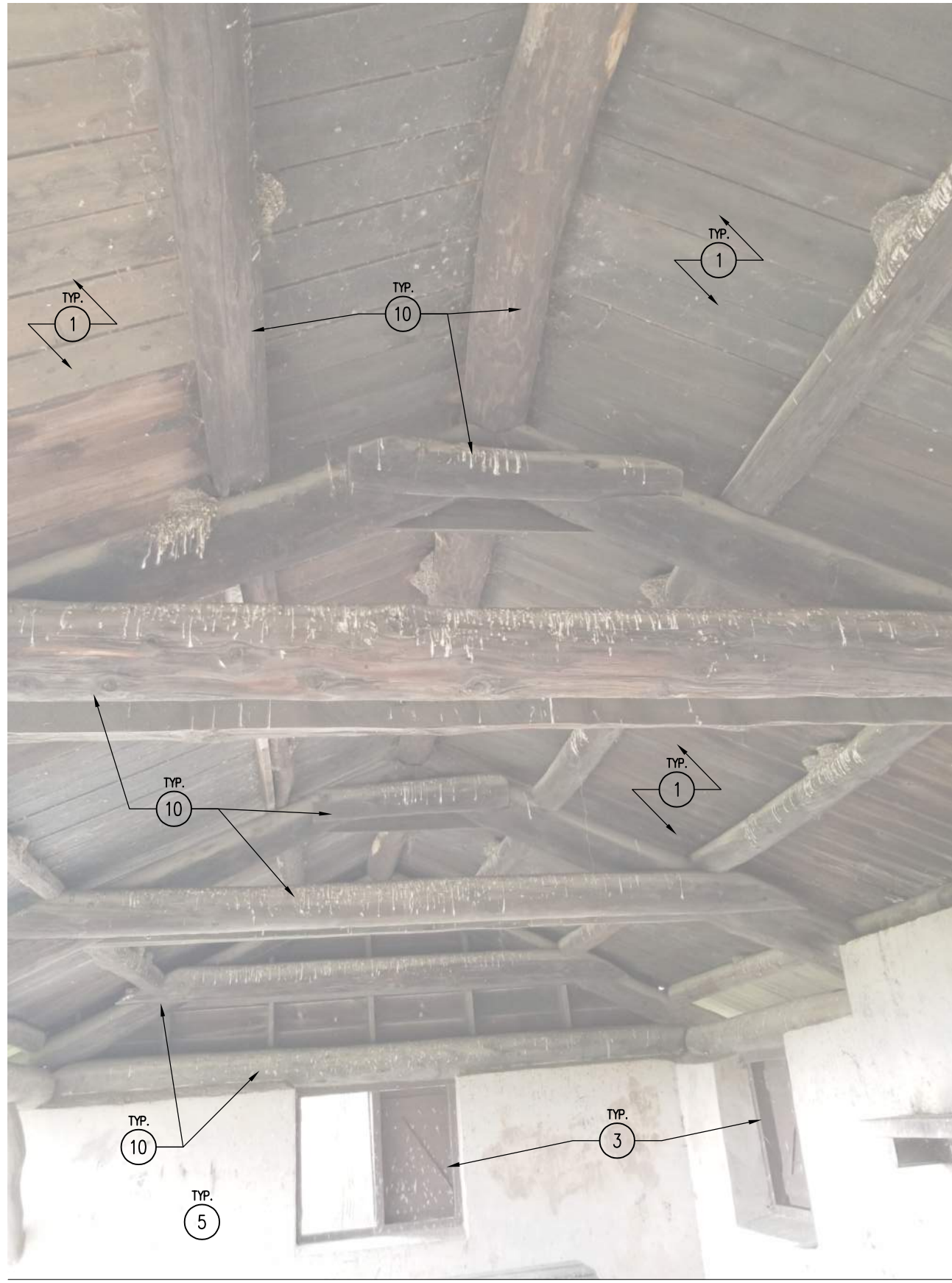
02 PHOTO – BEAMS, PURLINS, AND DECKING SCALE: NTS
