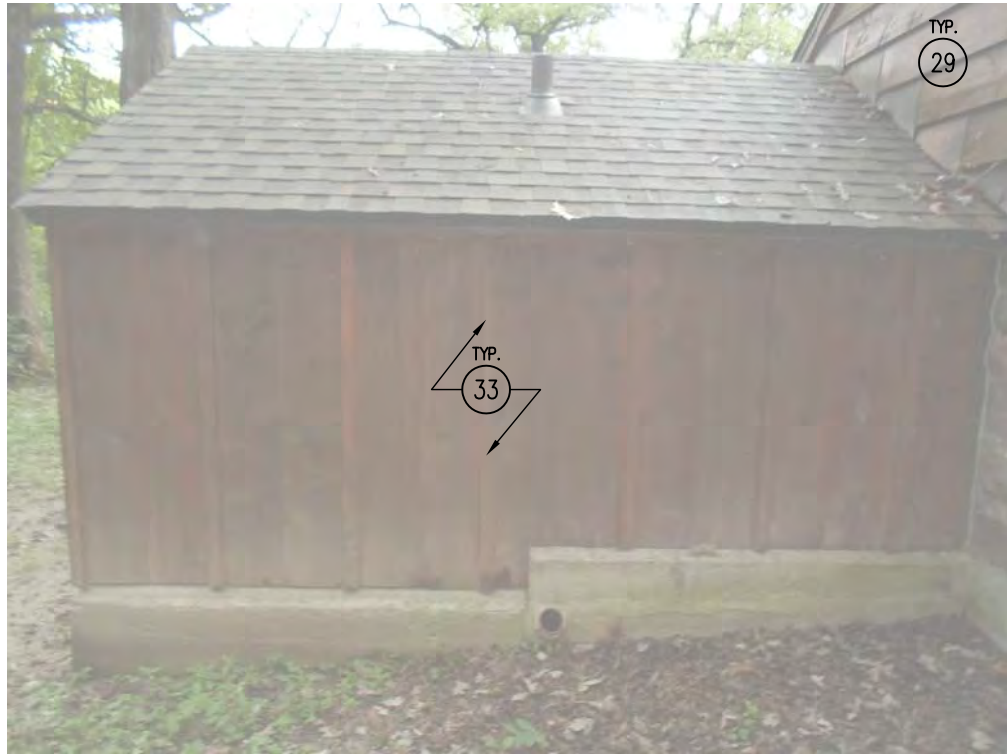
03 SHELTER PICTURE – SOUTH SCALE: NTS
