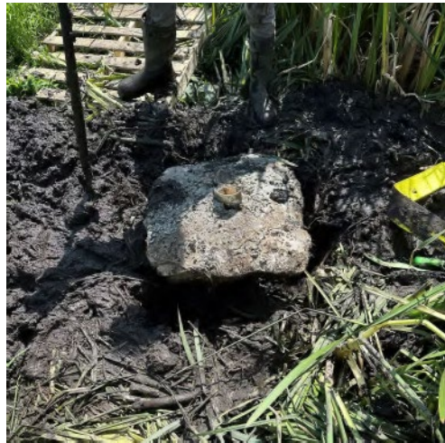
Photo 16: View of abandonment of WFE-7B.
