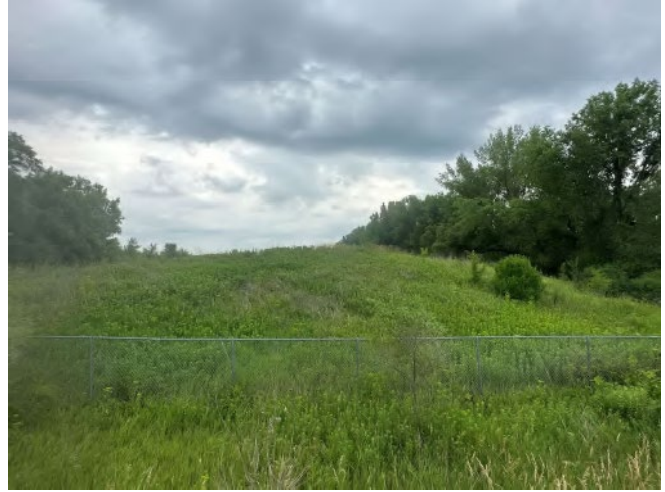
Photo 14: View of Northwest corner of landfill cap facing South.
