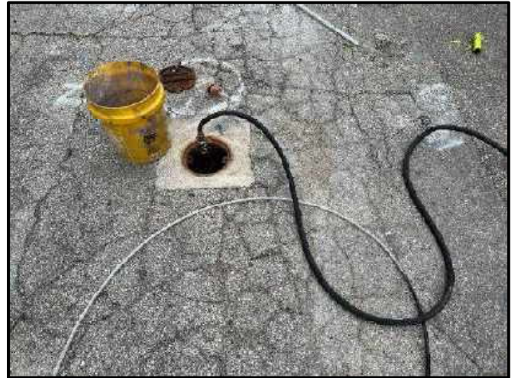
Photo 14: RRS attached an injection line to flush impacted monitoring wells
