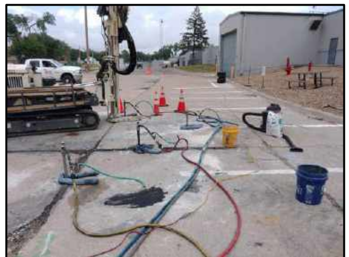
Photo 8: Active injection points in PFAS Pilot
