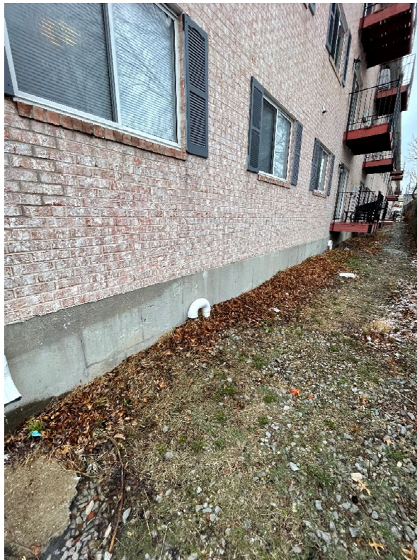
Photo 2: Louver on Site that is maintained and was observed free of debris during sample collection.
