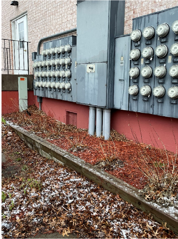
Photo 1: Observation of crawl space before sample collection.
