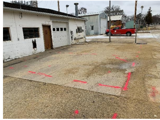
Area 2: showing potential piping in place.
