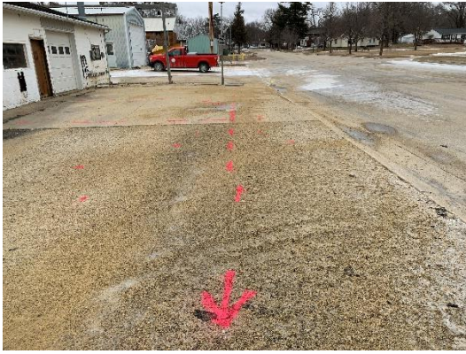
Area 2: showing storm sewer line.
