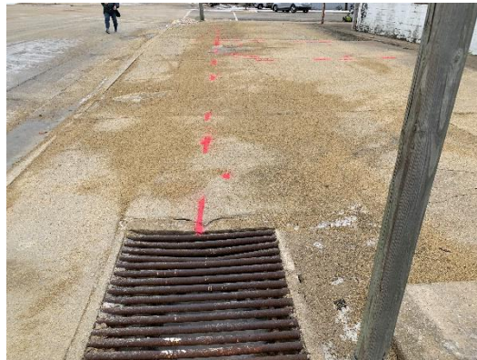
Area 2: showing storm sewer line and drain.
