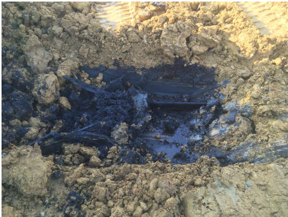
Photo 2 – Wooden box culvert near F5 with DNAPL residues (minimal free-phase NAPL). Was below 3' excavation but chased back under clean fill once identified. Blended with less impacted soils and transported under relief holder material manifest (facing west).
