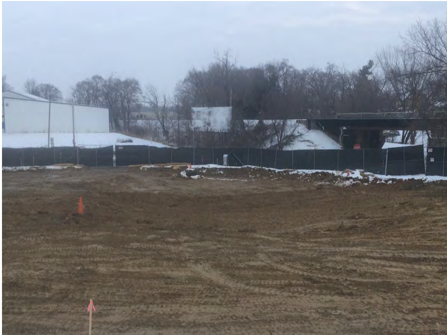
Photo 1 – View of southeastern portion of site where clean backfill is still several feet below original grade (facing SE).
