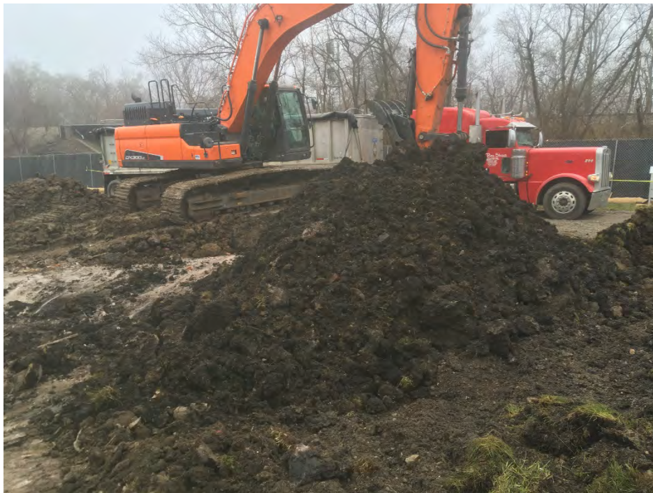
Photo 2 – Temporary stockpile of relief holder materials consolidated with less impacted waste soils at 1:6 ratio (about to be loaded for offsite disposal; facing SE).
