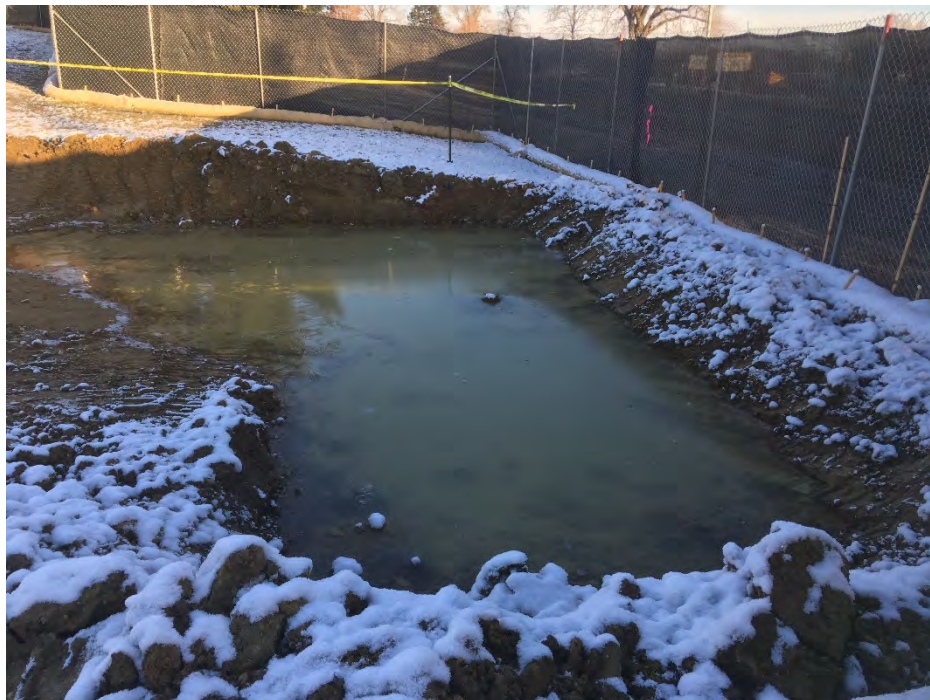
Photo 4 (Monday morning) – Pooled precipitation water in shallow excavation near J3; excavation had initial lift of clean backfill and berms prevented any flow of impacted water/sediment into this area (facing north). Water infiltrated surface (no run-off observed) in exclusion zones where minimal impacted material was exposed (perimeter of these areas also protected by wattles and clean fill berms).
