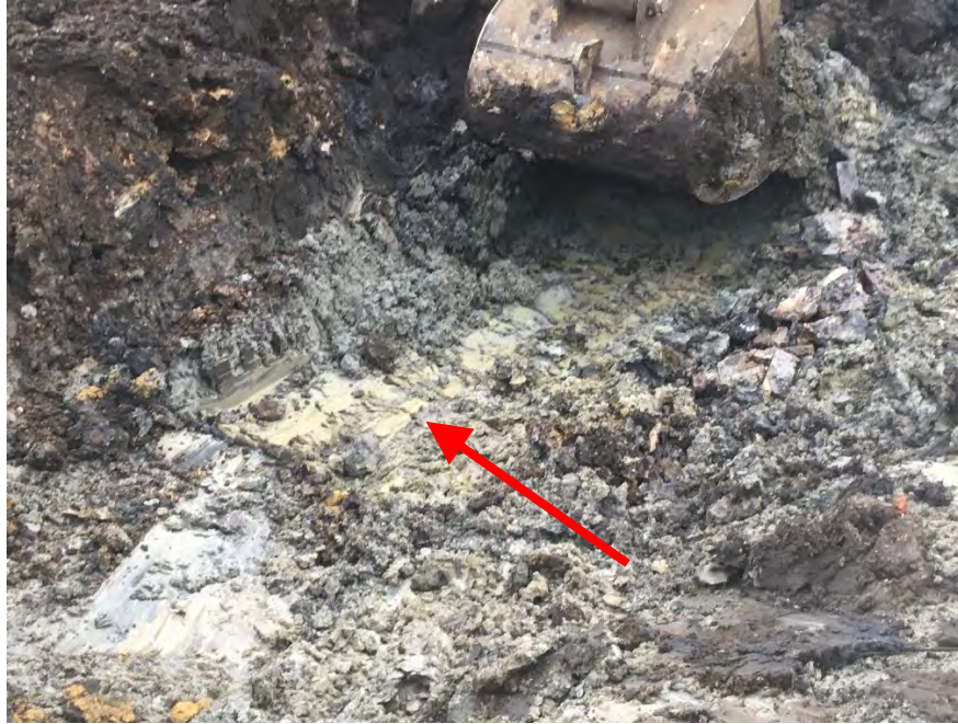
Photo 11 – Relatively clean native clays were encountered below DNAPL impacts (photo 10) at depth of approximately 7' bgs (facing SSE).
