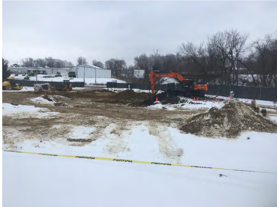
Photo 2 – View of site following bulk of snow removal activities (facing east).
