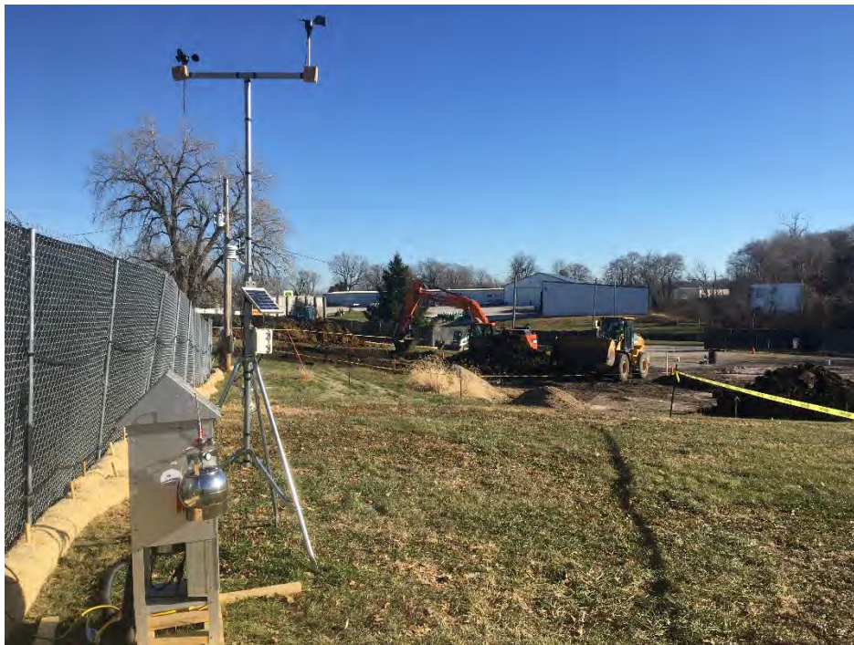
Photo 2 – Initial excavation of impacted materials along northern extent of excavation; air sampling and meteorological logging station in foreground (facing ENE).
