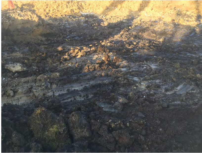
Photo 3 – Bottom of excavation near E8, with relatively minimal visual impacts at excavation depths of 1 to 3 feet (well shown in upper left corner; facing north).
