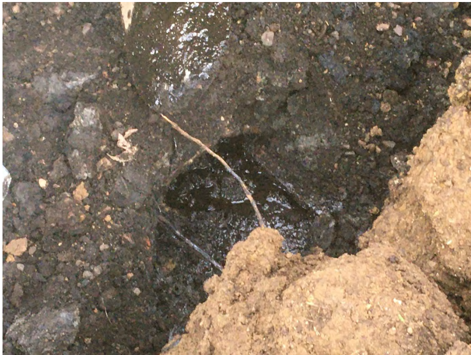
Photo 5 – One of three clay tiles encountered at approximately 2 to 3' below grade at eastern extent of excavation near J3/J4. All full of water with trace NAPL (heavy sheen), but no apparent flow. (facing SE).
