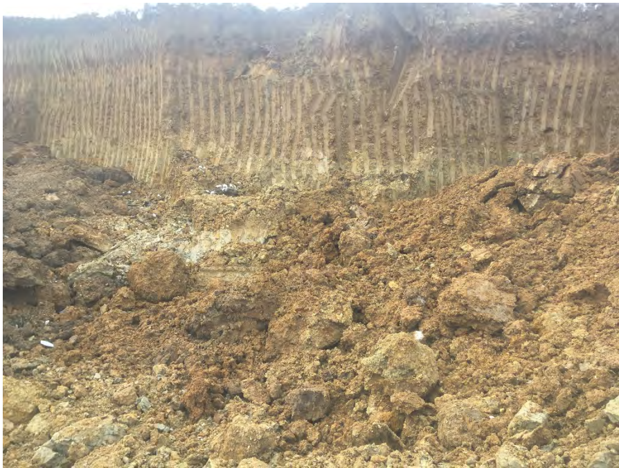
Photo 2 – Exposure of native clays at borrow area (facing west).
