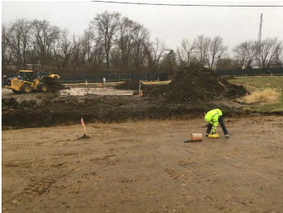
Photo 4 – Compaction testing near E3 (facing S).
