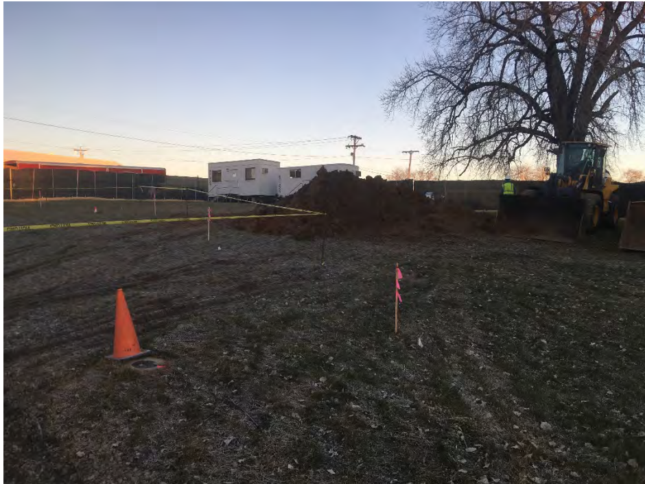
Photo 1 – Clean fill stockpile placed NE of excavation area (facing NW).
