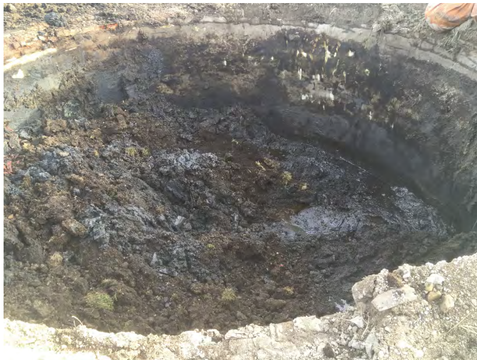
Photo 2 – View into relief holder – approximately 60% of contents have been excavated. Structure is made of standard size red brick with cement veneer interior (facing SE).
