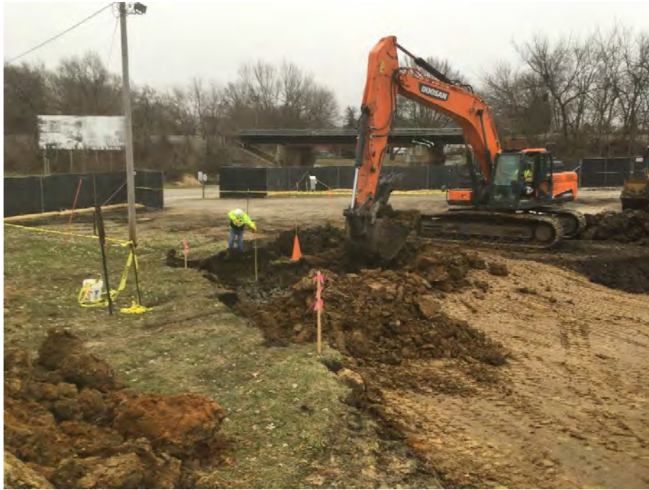
Photo 3 – Excavation near G3 on site grid (facing SE).
