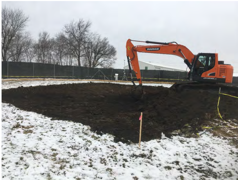
Photo 5 – Shallow excavation on Henderson property (facing NW).
