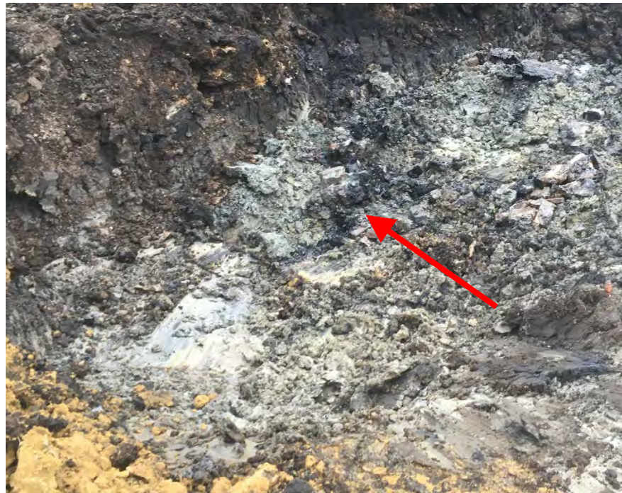
Photo 10 – As excavating impacts shown above, DNAPL (presumably from tile joint) was found directly to the south of photo above (facing SSE).
