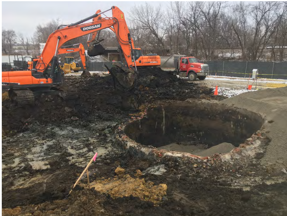
Photo 6 – Shallow excavation around NE corner of relief holder to depth of approximately 3 to 4 feet bgs and removal of holder wall to 3 feet bgs (facing SE).
