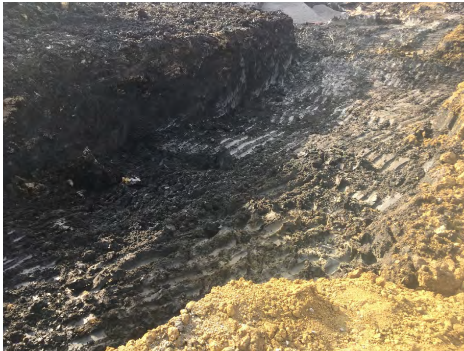
Photo 2 – Shallow impacts along north side of former building at depth of approximately 4 feet bgs. Right side of photo shows relatively less impacted clays (brown hues) while right side of photo shows more impacted blackish blue soil/mixed debris materials. Excavation on right side was extended to to about 7 feet bgs on far right side where brown hue clays were encountered (clean fill in foreground; facing SW).
