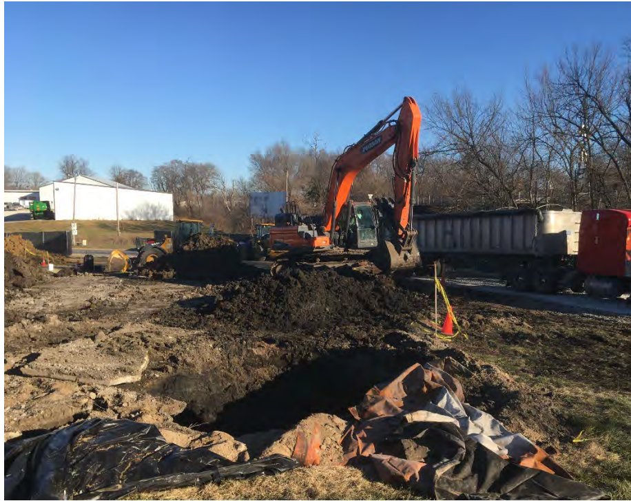
Photo 3 – Relief holder in foreground and consolidated stockpile in front of excavator about to be loaded. Aboveground stockpile limited to two truckloads at any one time, and covered with less impacted waste soil in between handling to reduce air impacts (facing east).
