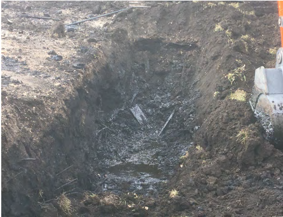
Photo 4 – Heavily impacted waste soils and wood debris in vicinity of I4. Excavation extended to approximately 8' deep at this location. Heavily impacted materials at this location consolidated with less impacted waste soils (facing west).
