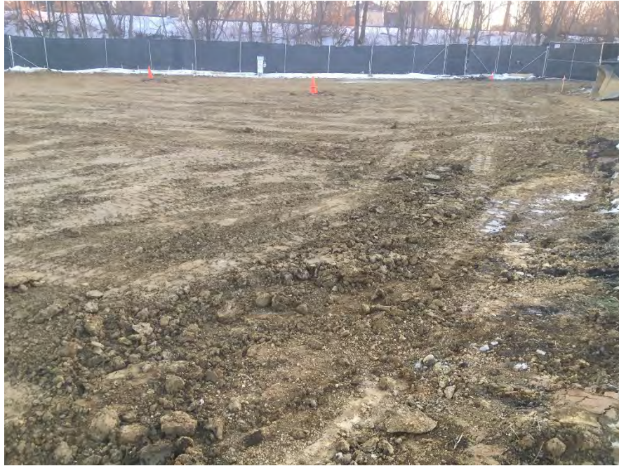
Photo 1 – View of backfilled excavation near where former building was located; backfill to approximately 0.5 feet below original grade (facing south).
