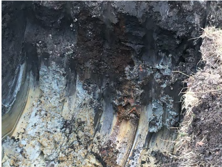
Photo 4 – Excavation of manway shown in photos 2 and 3, showing crushed tile that extended offsite toward the SE (facing SE). Wooden box culvert also found trending NE of manway (not shown).
