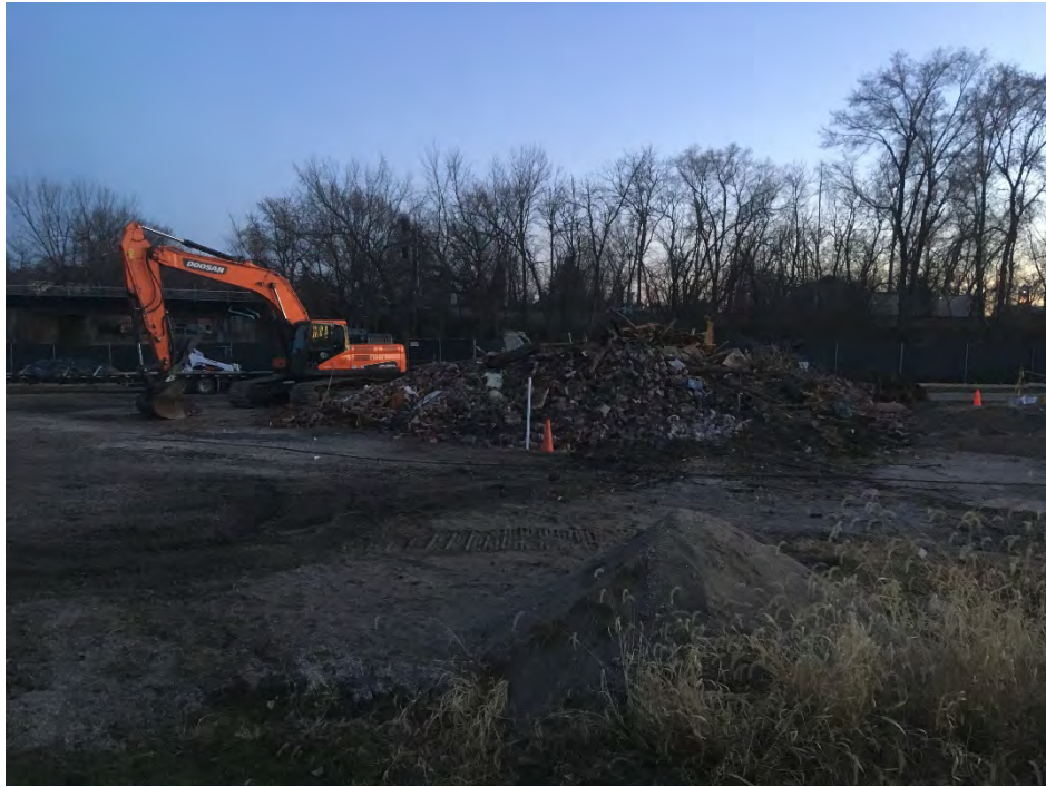
Photo 3 – Debris from building demolition (facing SE).
