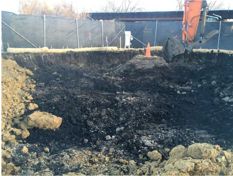
Photo 3 – Shallow excavation in southeast corner of site (facing SE).
