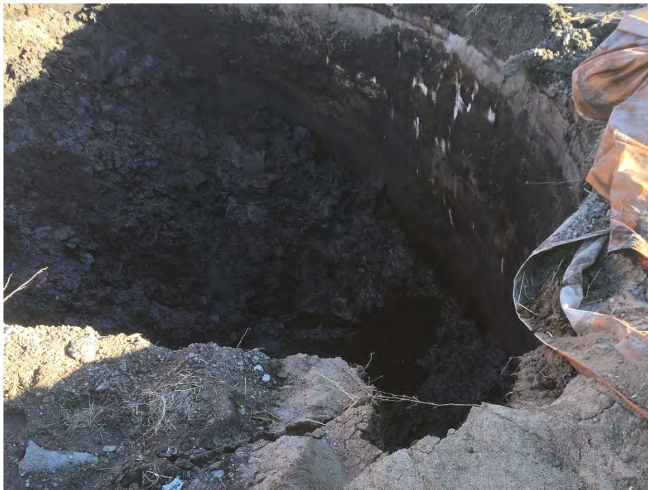
Photo 2 – View into relief holder – approximately 40% of contents have been excavated. Structure is made of standard size red brick with cement veneer interior (facing SE).
