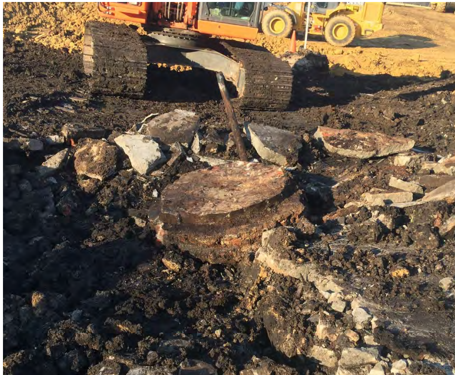
Photo 8 – Bottom of brick structure uncovered below former building floor on western half of building, east of holder. Structure remained together after repeated handling with excavator (facing NNE).
