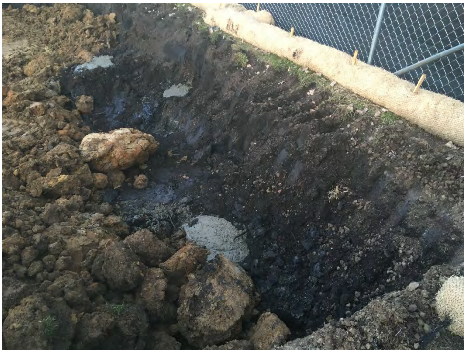
Photo 6 – Same three clay tiles sealed with concrete at eastern extent of excavation (buried fiber-optic utility just east of fence). Locations of all recorded with sub-foot accuracy GPS (facing NE).
