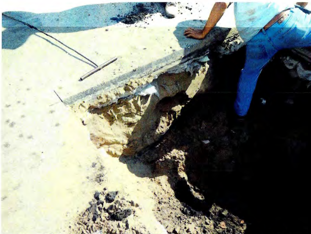
SE Excavation. Using prod rod to check sidewalls for USTs. Looking Northeast
