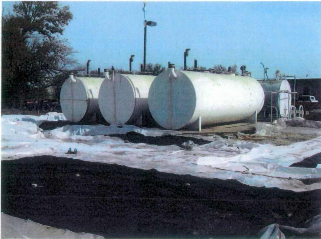
View is to the east of the above ground storage tanks (ASTs). Plastic cover was placed on the soil surrounding the concrete pad due to rain in the forecast.
