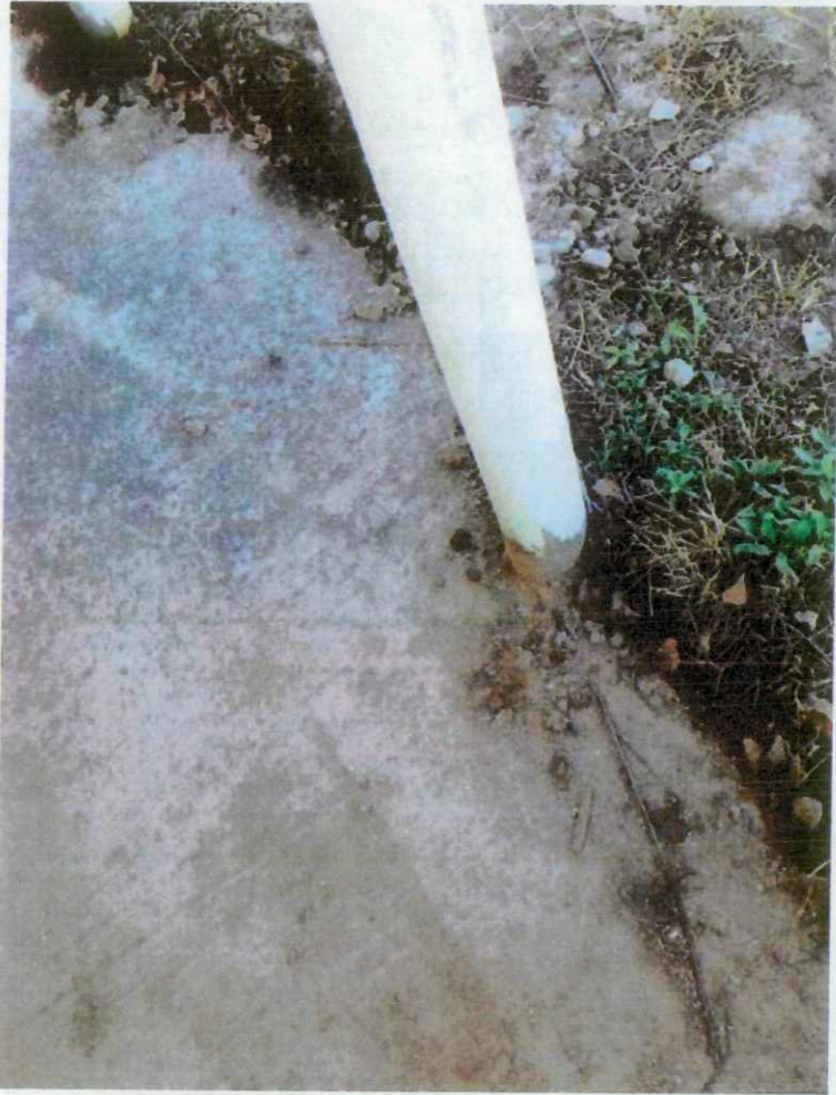
View is of the soil removed from under the fueling station.
