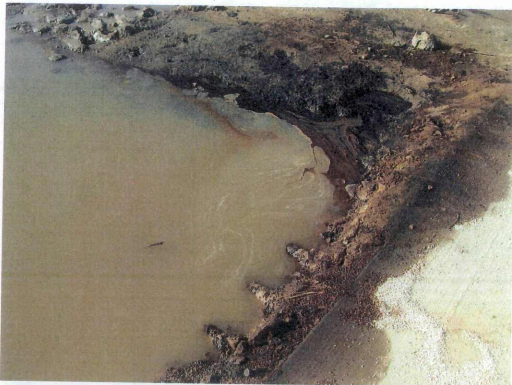
View is of the south side of the tank system after the plastic was removed. The concrete pad is visible to the right in this photo.
