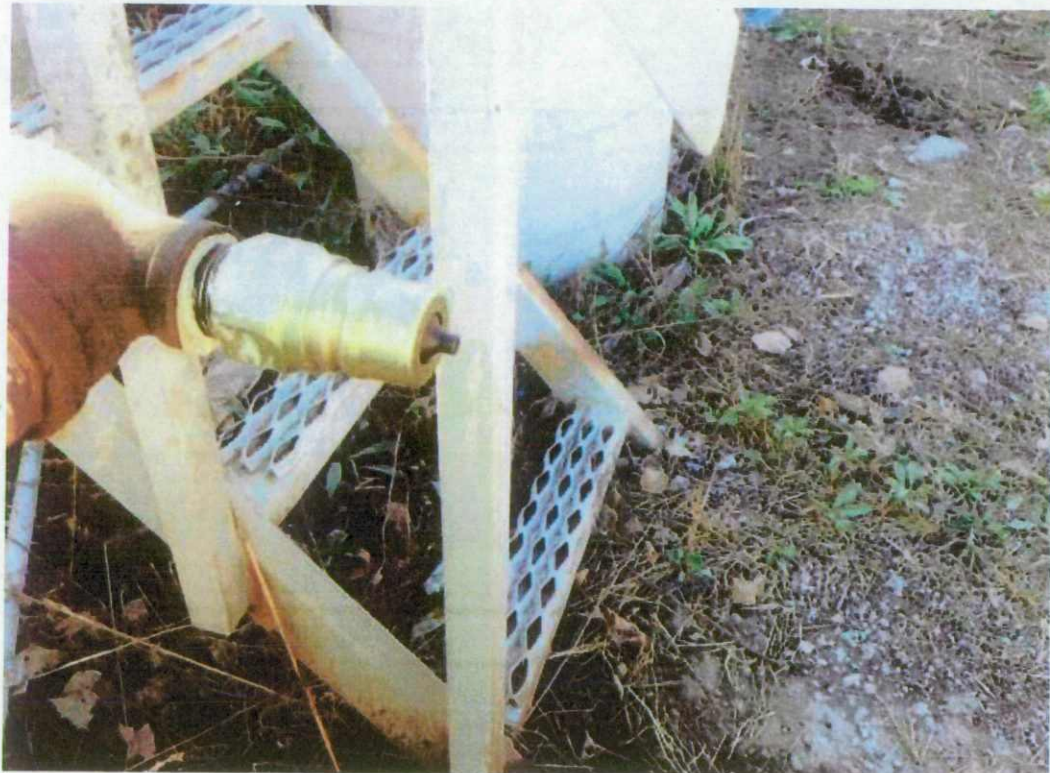
View is of the repaired pipe fitting at the fuel station.
