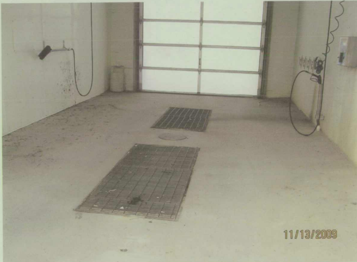
Photo 12. One of the wash bays located inside the original car wash. Grated floor pits are located in each wash bay.
