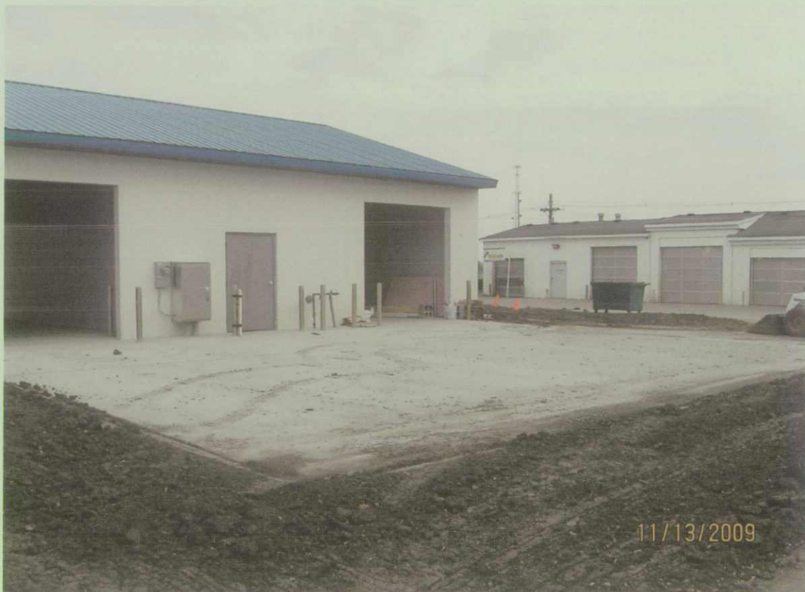
Photo 4. Northeast view of the subject property from the southwest corner showing the new car wash on the left and the original car wash on the right.
