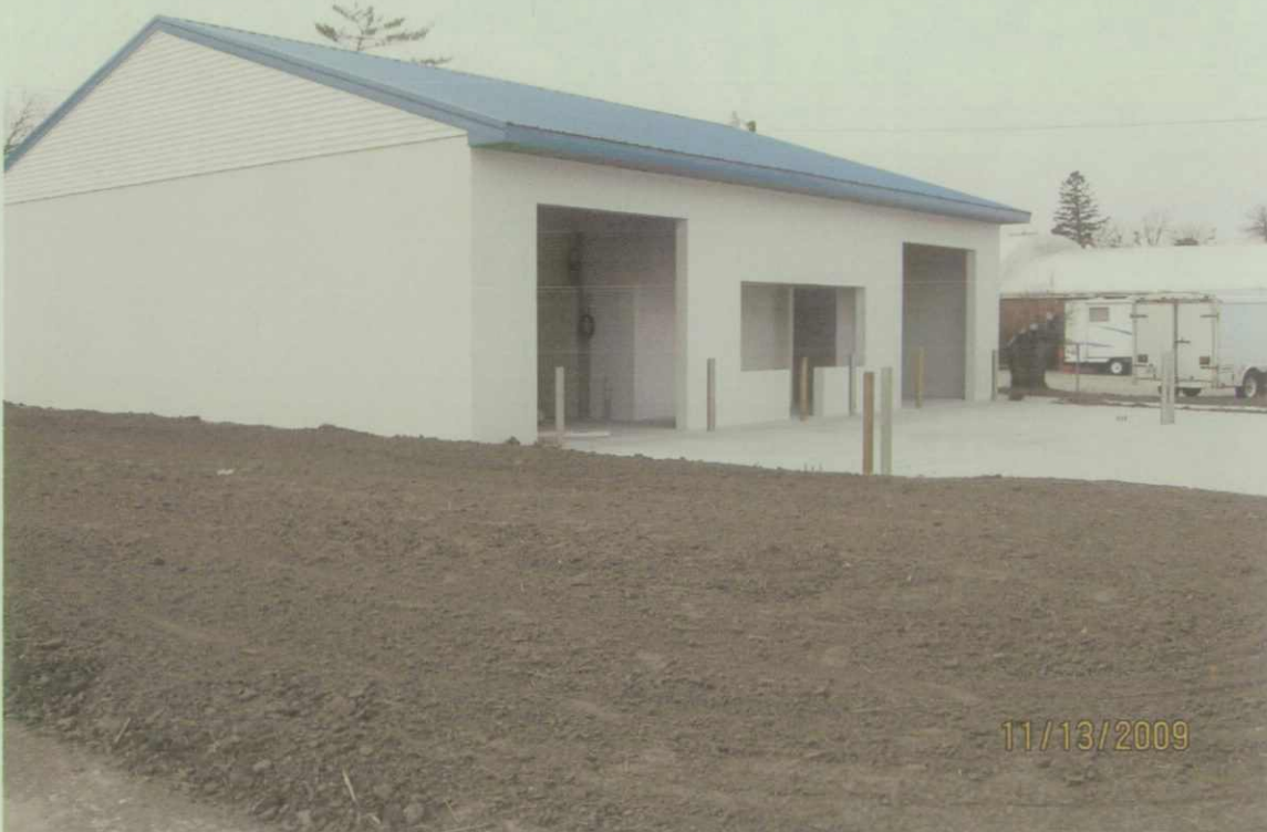
Photo 2. Southwest view of the new car wash located on the west side of the subject property at 1436 Lincoln Way.
