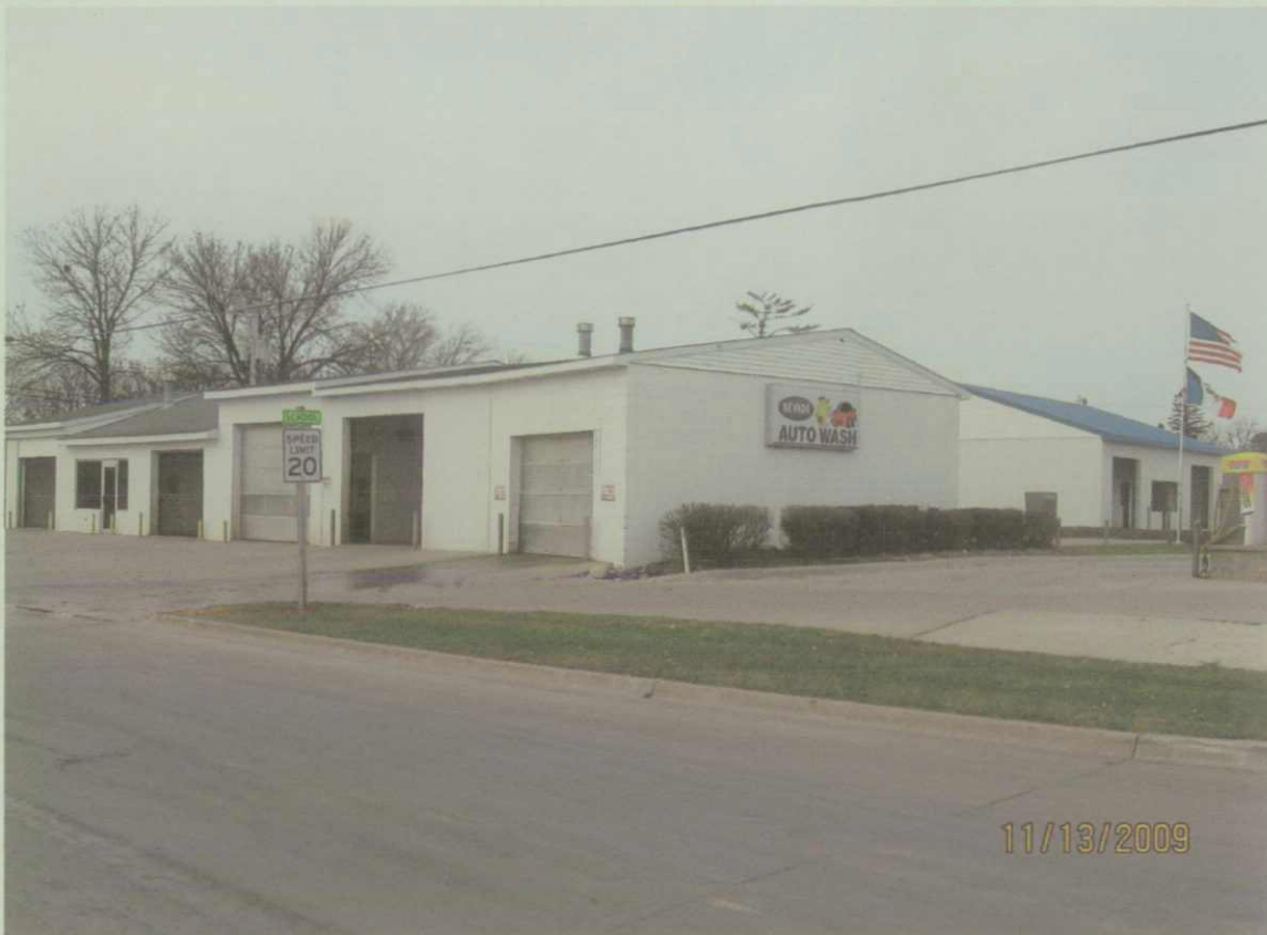
Photo 1. Southwest view of Nevada Auto Wash showing the 1120 15 th Street building on the left and the 1436 Lincoln Way building in the background on the right.
