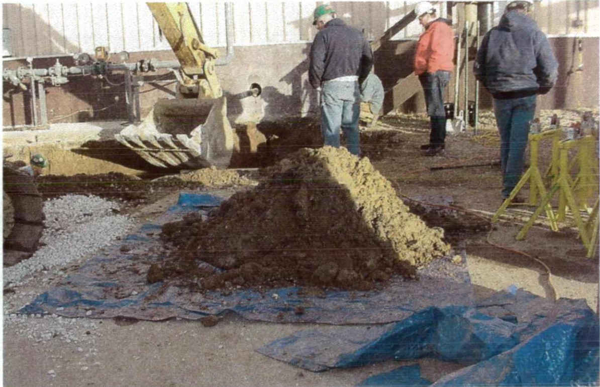
Figure 3- Segregated soil was placed on a plastic tarp and covered (photo taken facing North).
