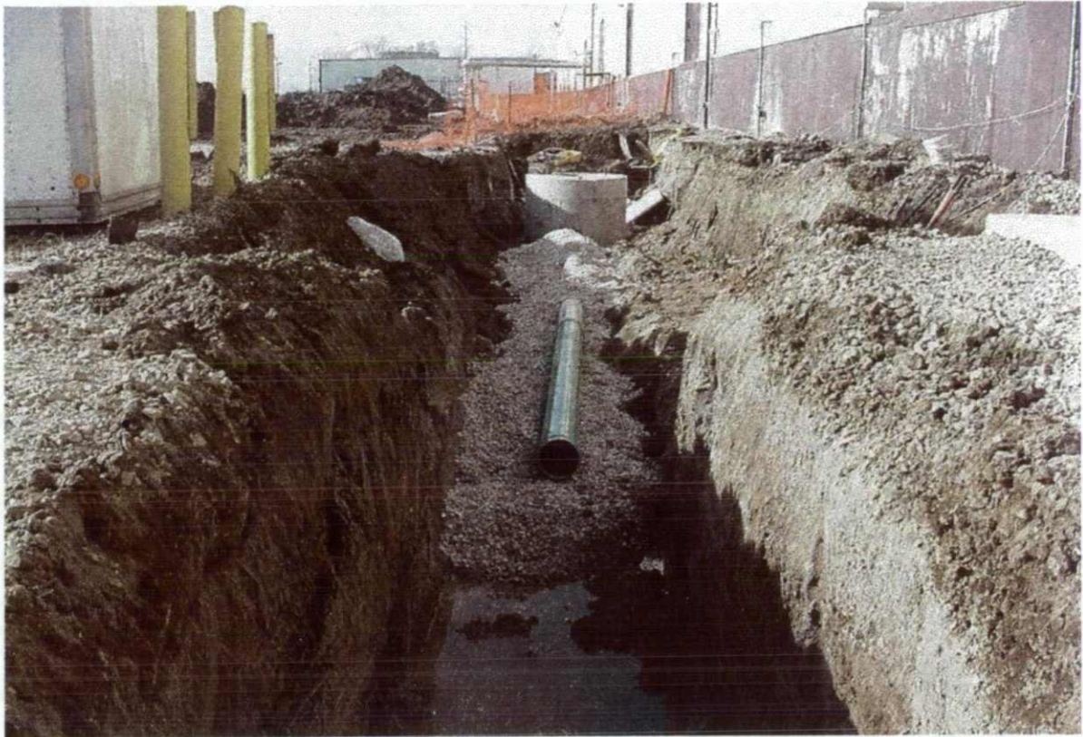
Figure 1- Overview of the sanitary sewer installation, showing the discolored soils on the left (photo taken facing West).
